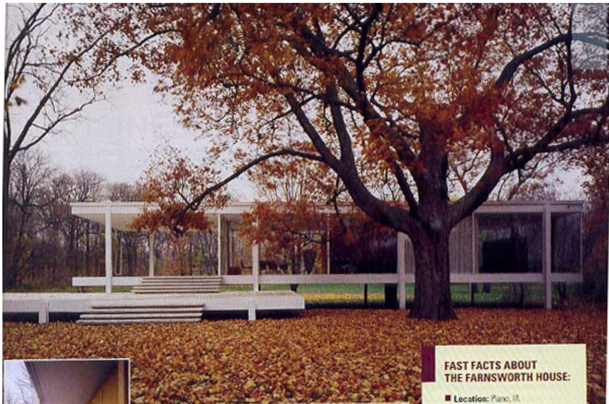
Eight steel piers arranged in three adjacent squares support the main building. A brass screen, now removed, once enclosed the upper porch to thwart insects.
