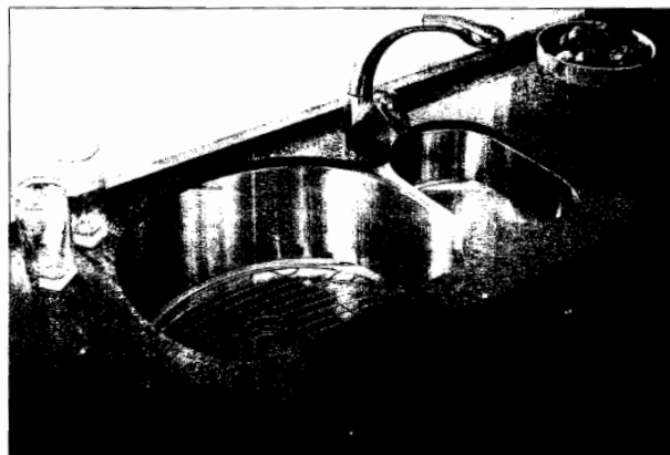
UNDER-MOUNT. Everyone, it seems, wants the clean lines and convenience that comes with under-mount sinks like the Kohler style above. With no lip, you can brush the crumbs on the counter right into the sink. The catch is under-counter sinks only work with a hard-surface countertop such as granite.
