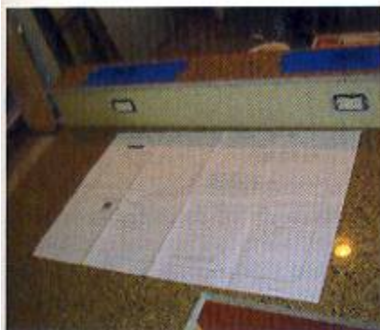
Here's a tough one in getting the outlets right between a base and a snack bar. It took some pre-planning (left) and a good on-site cut (middle) to get the job done right. (Right) Here's another one done on a Caesarstone® splash between a base and a snack top.
