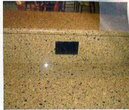
Here's a tough one in getting the outlets right between a base and a snack bar. It took some pre-planning (left) and a good on-site cut (middle) to get the job done right. (Right) Here's another one done on a Caesarstone® splash between a base and a snack top.
